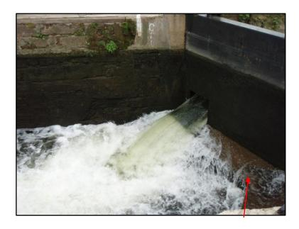
A gate paddle fully open showing the force of water that can enter the lock chamber. The cill can be seen on the right hand side at the base of the gate
