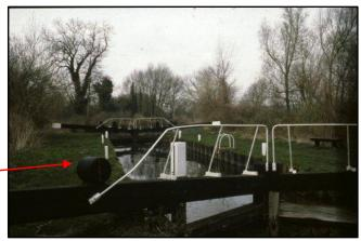
It is important to be aware of the position of the cill as boats need to be kept clear when the lock is being emptied otherwise the stern of the boat could be caught on the cill eventually severely damaging the boat as the water level falls
